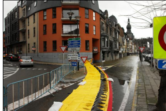
Figure 14 : Protection inondation souple ( https://www.megasecureurope.com/?gad_source=1&gclid=CjwKCAjw59q2BhBOEiwAKc0ijfOCyJozjsFXr4EjbJpXUixn4GyZ-Y-H7_44cmeRuamwqG8W8LDhwxc0ze4QAvD_BwE ).
